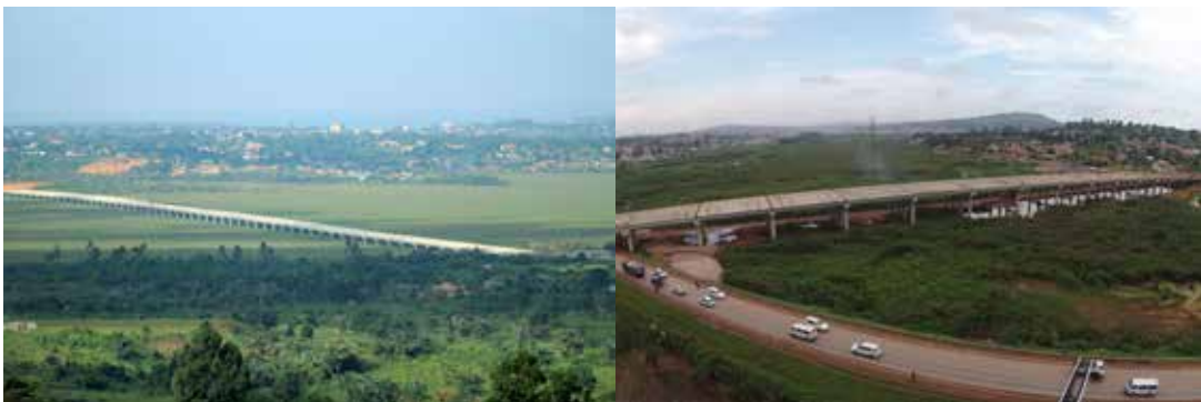
Kampala Entebbe Express Highway (Photo credit: UNRA)
