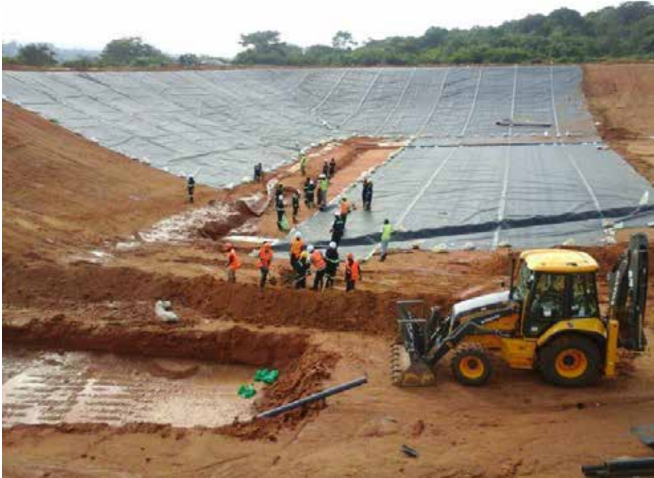
Construction of hazardous waste landfill in Hoima (Photo credit: NEMA, 2014)
