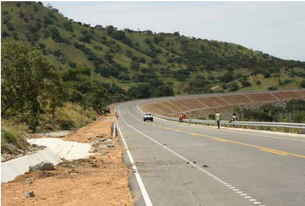
The new Hoima- Kaiso Tonya Road (Photo credit: John Diisi, NFA)
