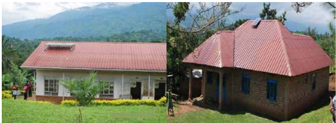
Solar panel installation at Bumadu Seed S.S. in Bundibugyo (right), and a home in Kibiito with an installed solar system under REA's PVTMA (left) (Photo credit: MEMD 2014)
